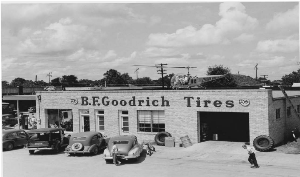
Before the Bell could make a splashy rooftop landing in Rosenberg, the building had to be shored up with beams hauled from a lumberyard by mule teams. (LBJ Library)
