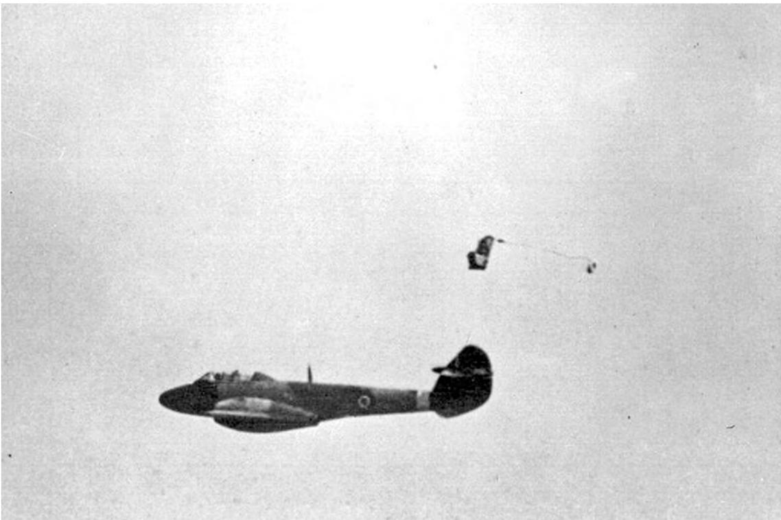
***Lynch makes the first live ejection from a Meteor at 320 mph and an altitude of 8,000 ft. on July 24, 1946. Credit: Martin-Baker***
