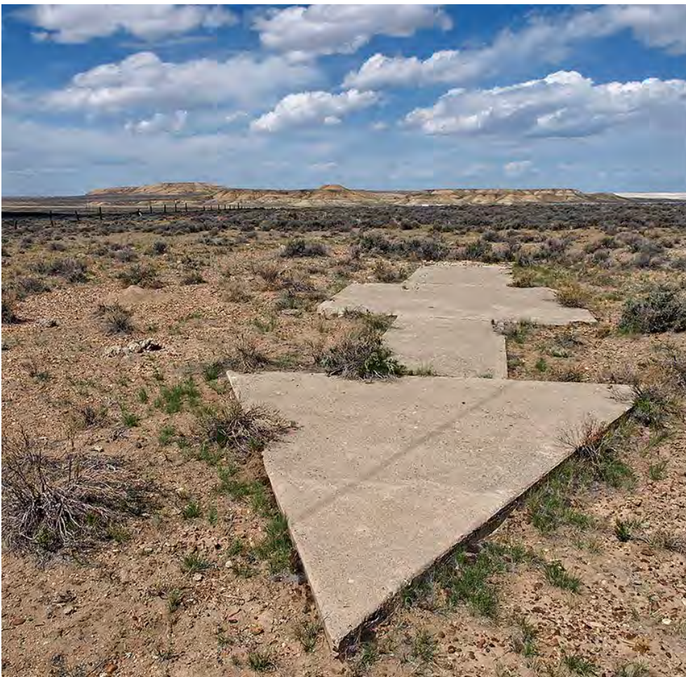
Many of the arrows built in the 1920s to guide airmail pilots are still in good shape, like this one in Sweetwater County, Wyoming. (© dreamsmithphotos.com)
