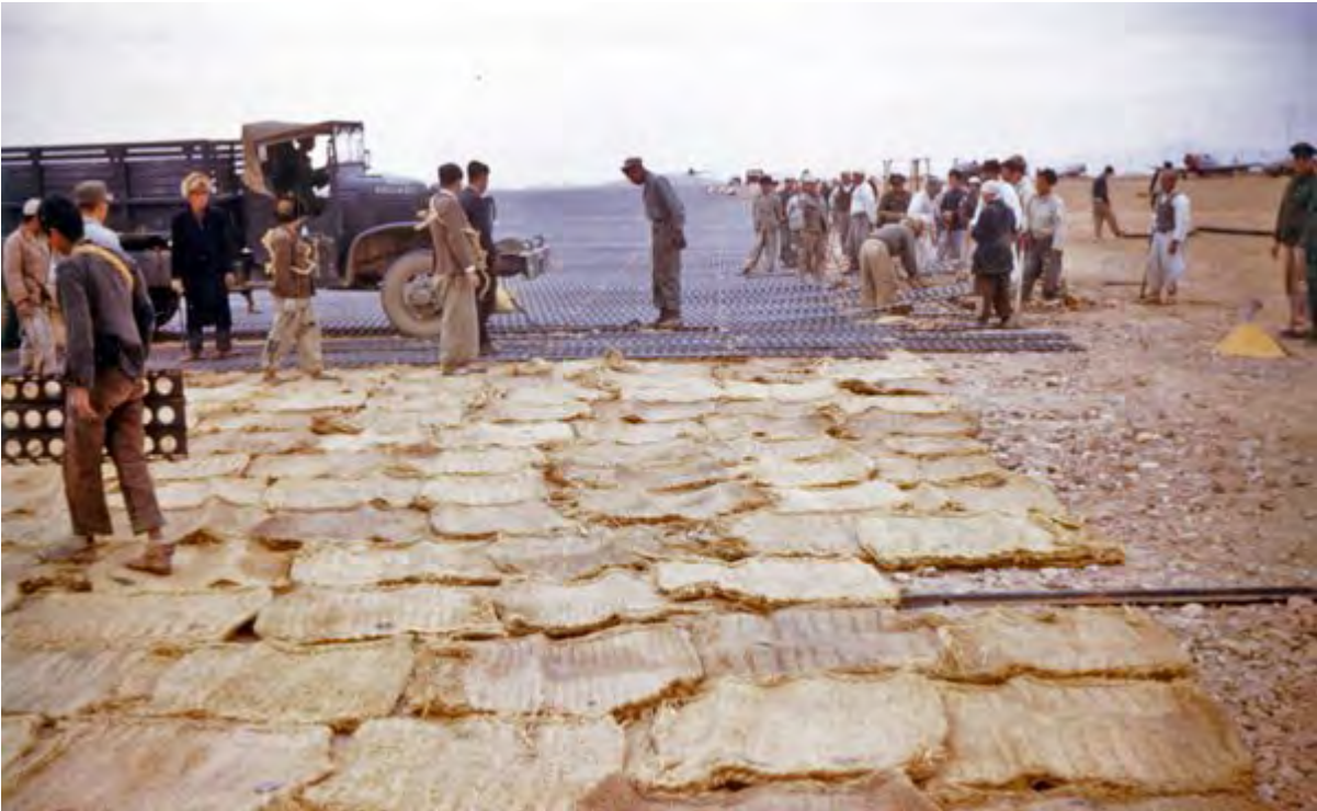
Most U.S.-built runways at Korean bases such as this one—field K-6 at Pyongtaek—were made of PSP. Steel mats were often laid over vegetation or straw, or in this case rice sacks, to help drainage and reduce dust.(USAF)
