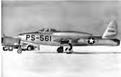
Republic P-84B; note the small engine air-intake in the nose. (USAF Photo)
