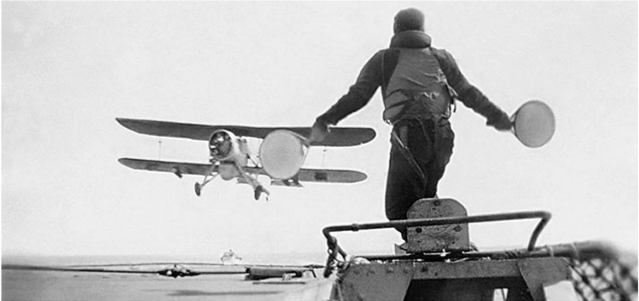
Called "Bats" after the disks he used to signal pilots, a landing officer says "Lower!" to an approaching airman. The air-to-surface vessel radar dome is visible between the airplane's gear struts.
